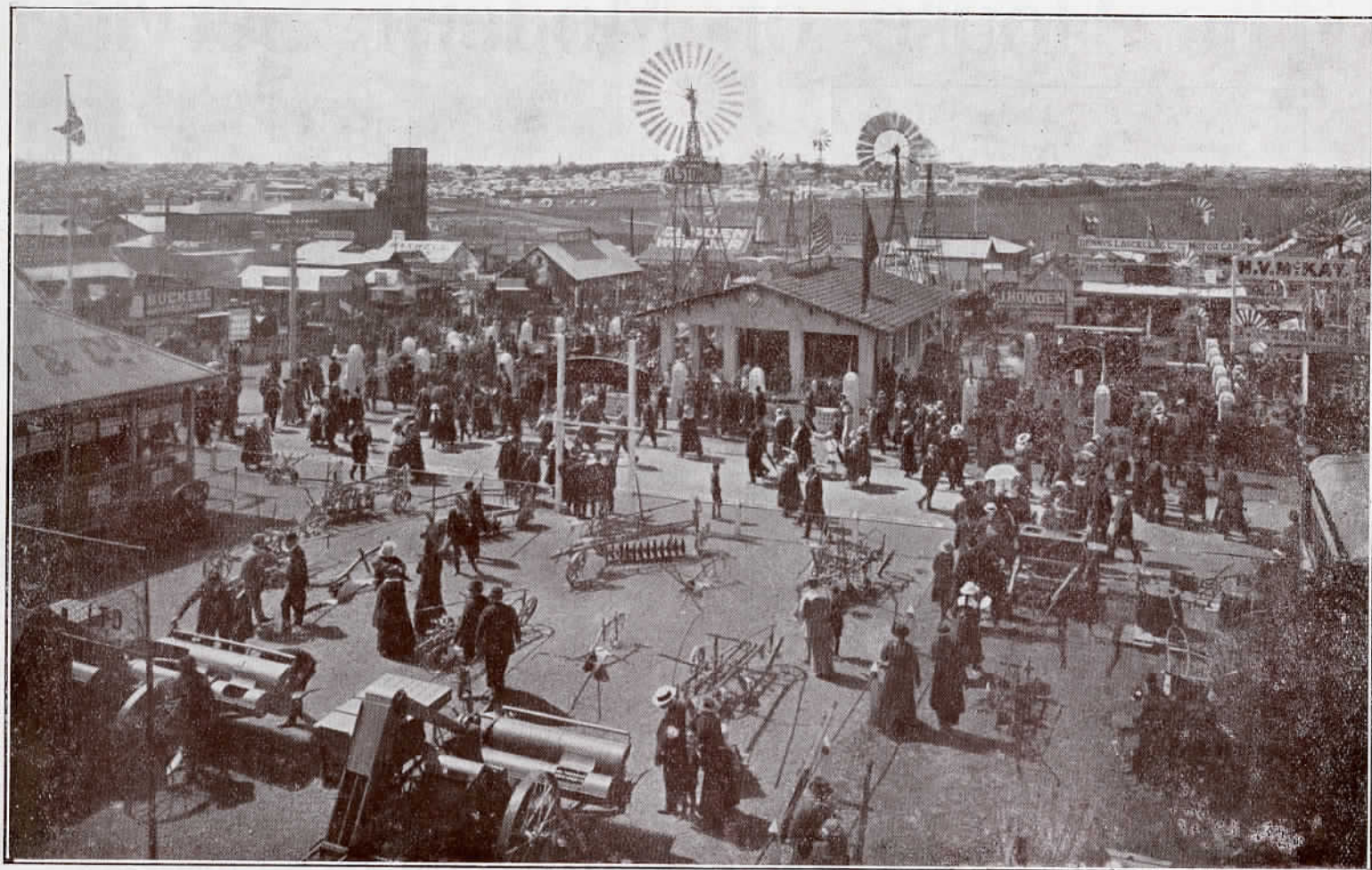
General View New Machinery Court.
