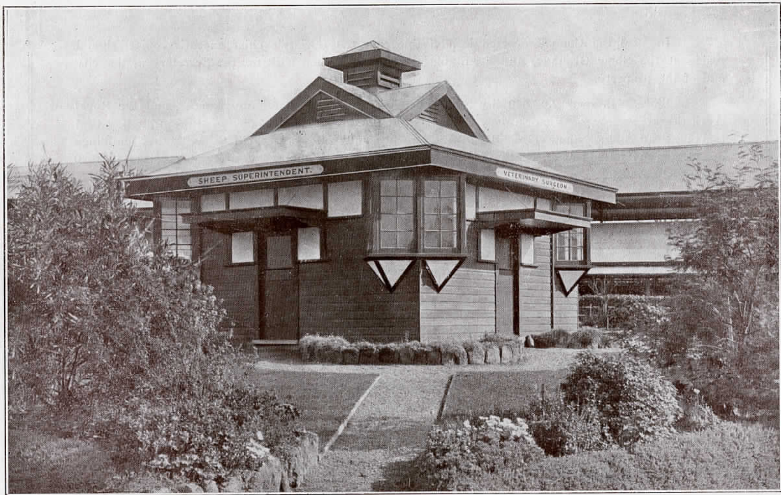
Superintendents' and Veterinary Surgeon's Offices. Erected 1919.
