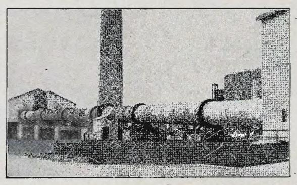
Large Rotary Kiln at Cement Works, Fyansford, Geelong
