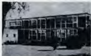
The Science Wing completed in 1974 contains three Laboratories, Preparation Rooms and a Mathematics centre.
